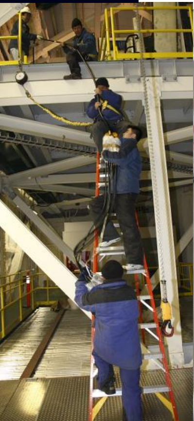
Fibre cable installation
